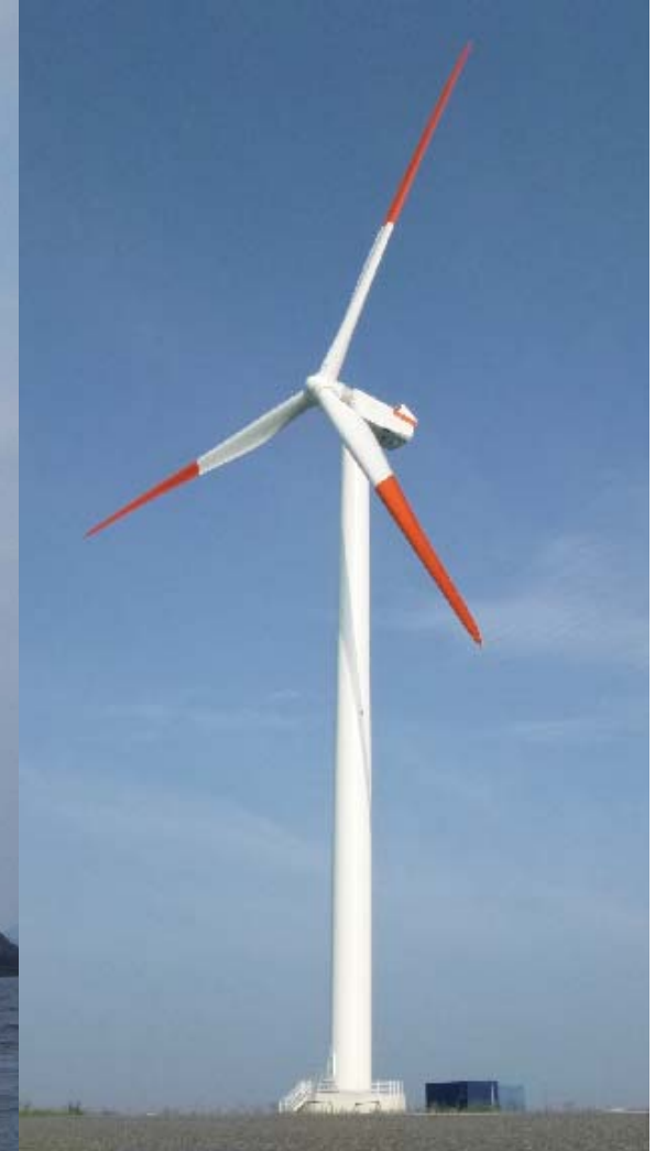
Japan Steel Works (JSW) 2.7MW, gearlessPMSG
