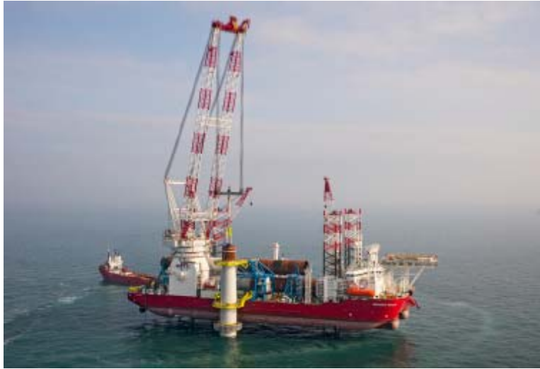
Scylla installing the world's largest MP
